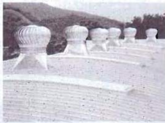
Extractores de aires
