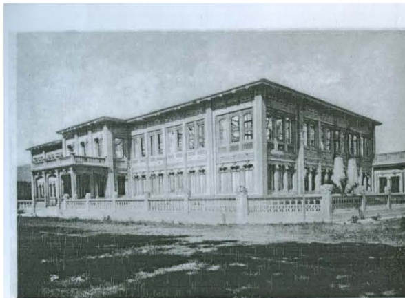
Escuela Normal en construcción San Salvador High-School during construction
