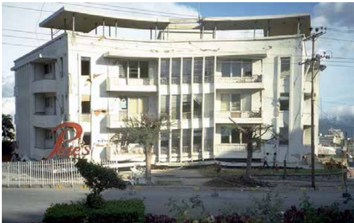
Figura 134. Daños observados durante el sismo de 1986, M5.7 – San Salvador 61 Fuente: Olson, Robert A. Collection. Earthquake Engineering Online Archive, National Information Service for Earthquake Engineering, EERC, University of California, Berkeley
