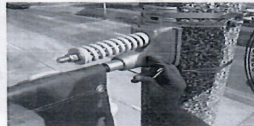
step 4 Insert zip tie through banner grommet and pin.
