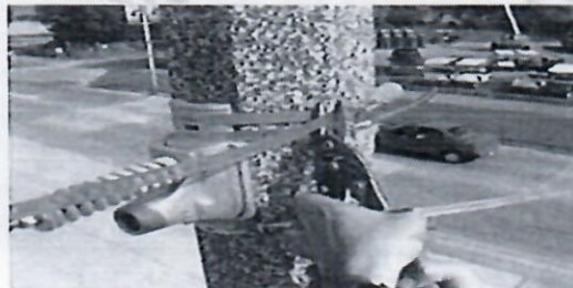
step 3 Install fiberglass arm and insert pin into nose.
